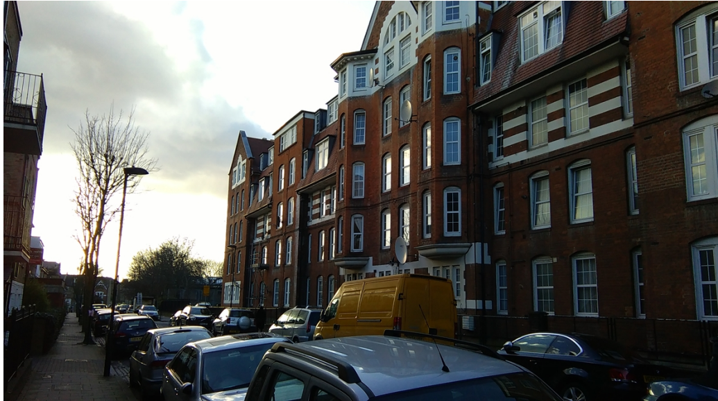
Photograph 3: View of estate from Wedmore Street looking north
