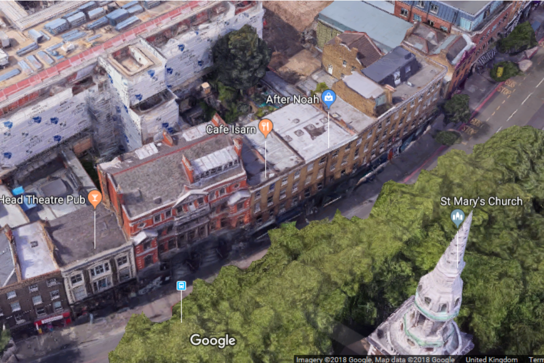
Figure 4: Site viewed from the north looking onto the flat roof of the King's Head
